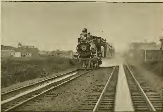
DOUBLE TRACKS AND TANKS (N. Y. & L. H. RAILROAD) NEAR LONG BEACH, N. J. ENGINE NO. 6010. WATER RISING 25 FEET PER HOUR.
